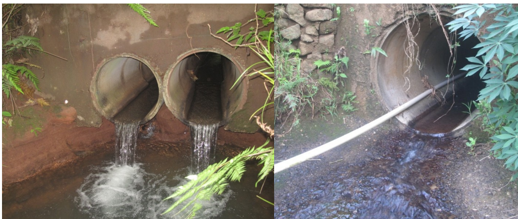
Above left: Hanging culverts near Nabalabalawa, giving no chance for fish to climb upstream. Above right: Culvert with fish ladder (rough concrete surface in front of culvert) to help fish with their upstream migrations.
